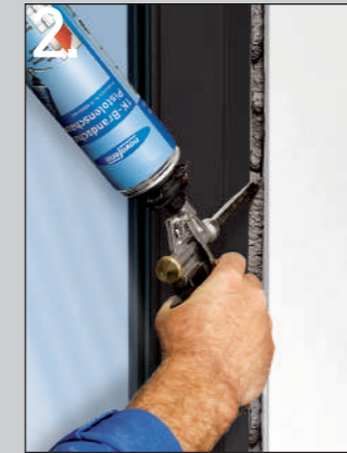
2. ... fill with fire protection foam...
