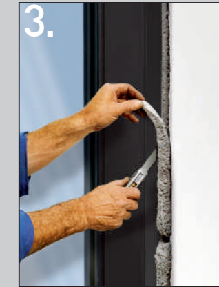
3. ... remove excess foam once dry...
