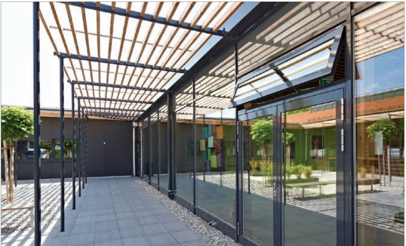
GEZE OL 90 top-hung, outward opening, Stiftung Ecksberg, Mühlendorf, Germany (Photo: Robert Sprang)
