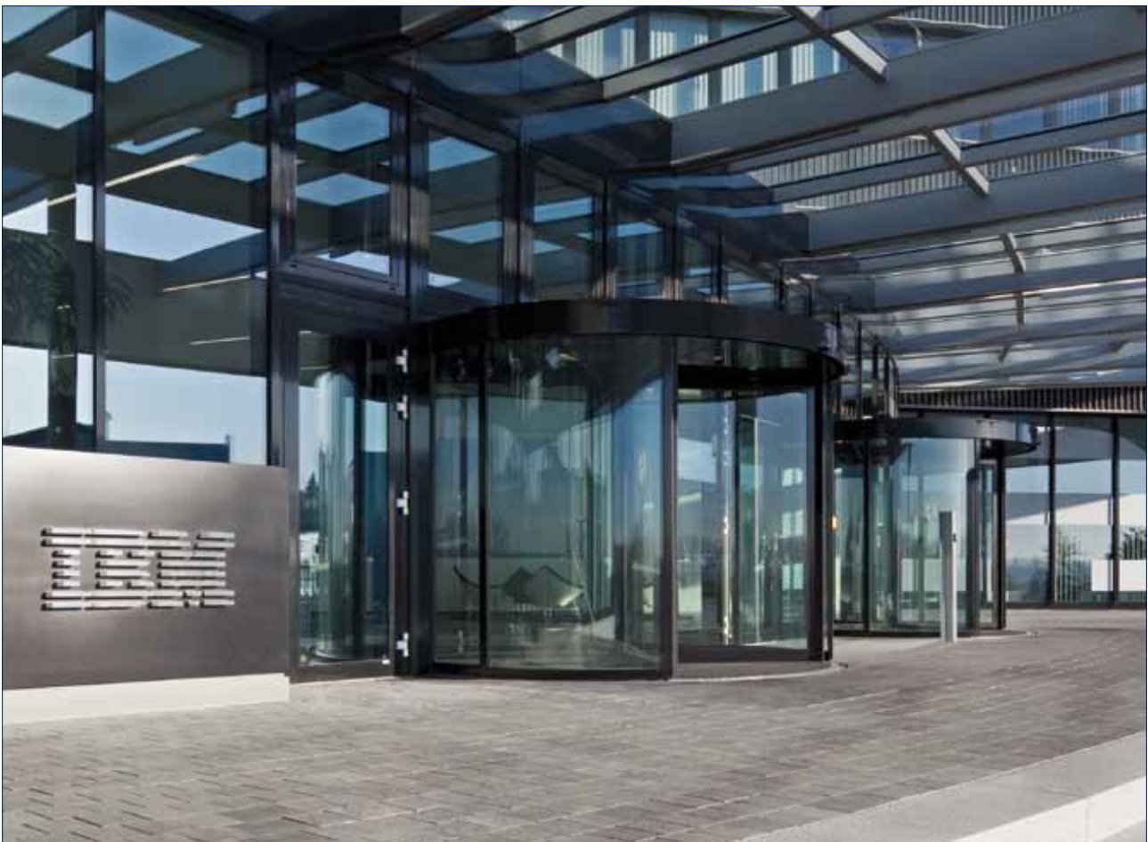
IBM Ehningen - Fully-automatic GEZE revolving doors with 4 leaves, BO function and automatic night time locking mechanism
